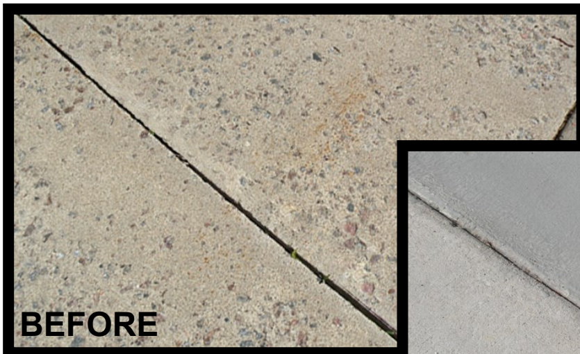
SPALLING CONCRETE
