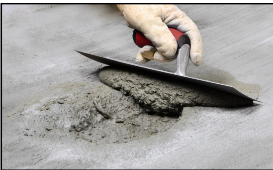
Example 1: Repair deeper blemishes with Rapid Patch®
