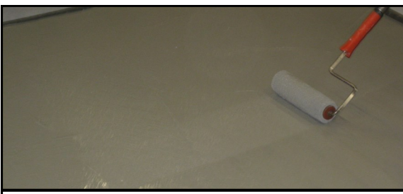
Example 4: Apply sealer using a roller
