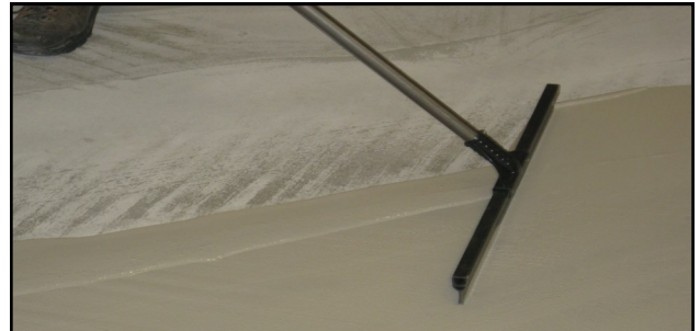
Example 2: Apply Akonakote® using a stiff-edge blade
