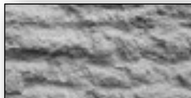
CSP 9 (heavy scarification)
