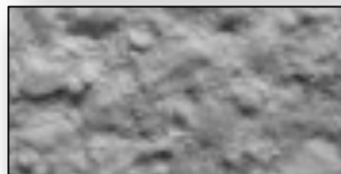
CSP 7 (heavy abrasive blast)
