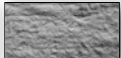
CSP 6 (medium scarification)
