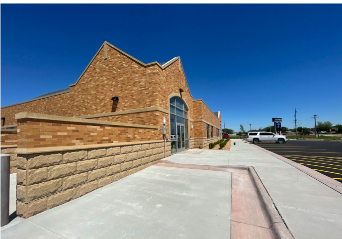
Sanford Clinic: Stone Mason Unit (Limerock)
