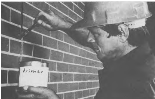
Proper priming of joint. (SWRI)
