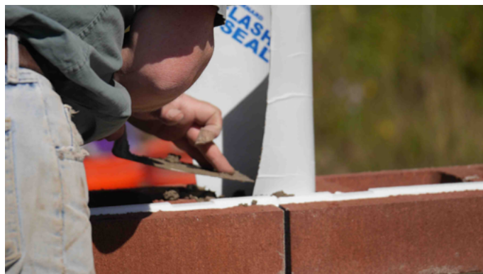
Bond break at control joint
