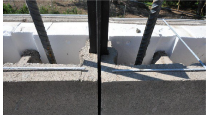
Control joint using HI-R-H Sash/Jamb Unit
