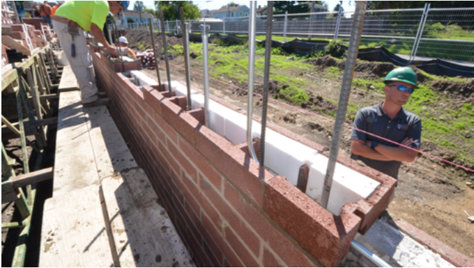
Jambs being constructed using HI-R-H Half High Sash/Jamb Unit
