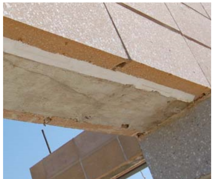
HI-R unit reinforced as lintel after grout has cured and wood forms have been removed
