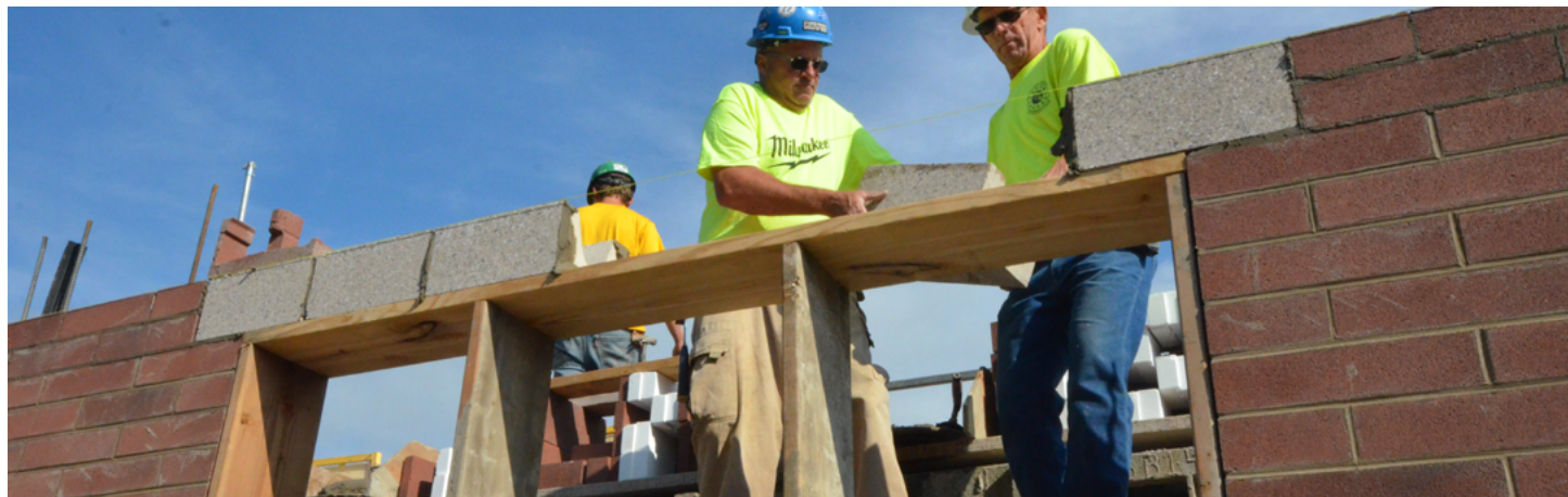
Traditional masonry lintel installation using a form (this lintel is not insulated)
