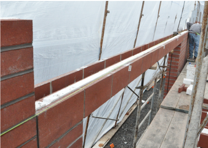
HI-R/ HI-R-H Closed Bottom Lintel Pre-fabricated installation
