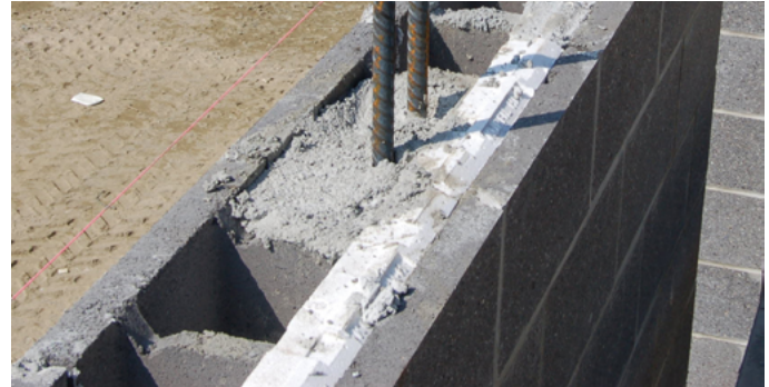
Partially Grouted HI-R Wall
