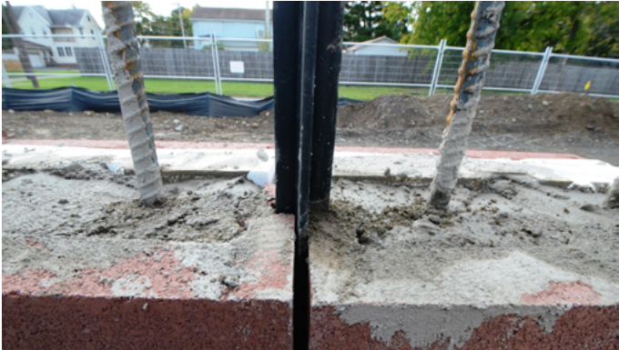
Control Joint using HI-R-H Half High Sash/Jamb Unit
