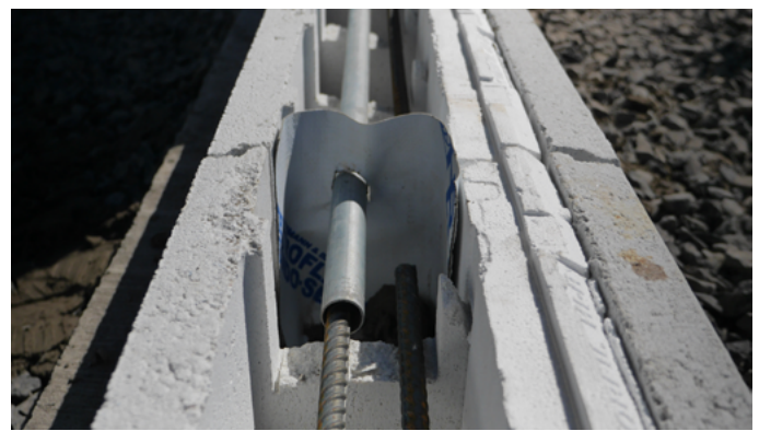
Bond break at control joint
