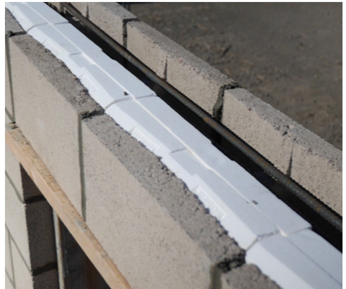
HI-R-H units reinforced as a lintel before placement of succeeding courses
