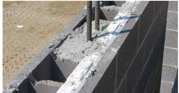
Partially Grouted HI-R Wall (shown with 12×8×16 unit)
