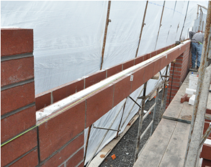
HI-R/HI-R-H Closed Bottom Lintel – Pre-fabricated installation
