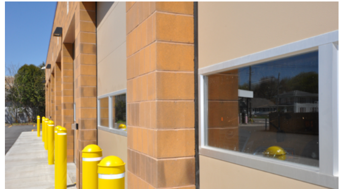
Finished Door Jamb using HI-R-H Sash/Jamb Unit
