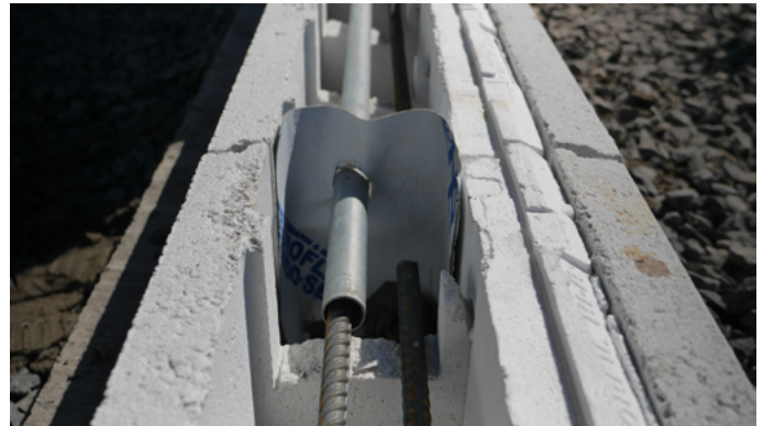
Bond break at Control Joint
