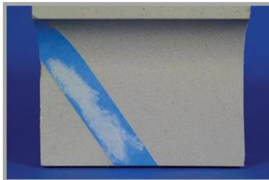
**STEP 4** – Shave the Matrix with a miter rod or edge of trowel to final form. Finish the repair to match the existing surface of terra cotta. In this case, the repair was finished smooth.
