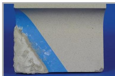
**STEP 3** – Apply the color matched Matrix to the repair zone. Over build and allow to 'set' until thumbprint.
