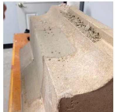
12. Finish - begin final finish of repair when mortar achieves preliminary set. Mortar will have rough scraping sound and will not stick to screed tool.
