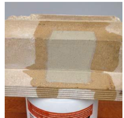
15. Cure - mist the repair (in hotter conditions) and keep adjacent substrate moist to maintain curing process within the mortar. Continue curing for 24-72 hours after installation.
