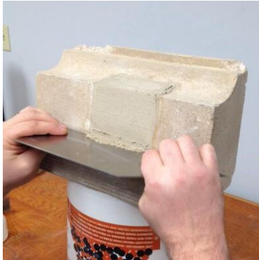
10. Pre-Screed - screed the patching mortar to within 1/4" of the final surface profile. Check for low spots.
