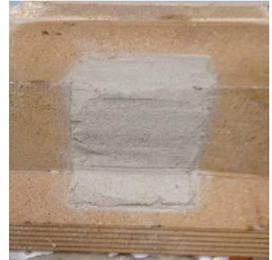
12. Finish - begin final finish of repair when mortar achieves preliminary set. Mortar will have rough scraping sound and will not stick to screed tool.
