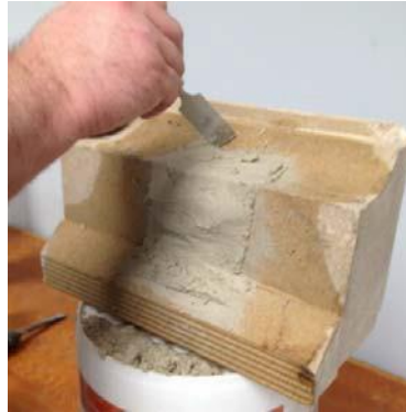
11. Remove heavy mortar smears.
