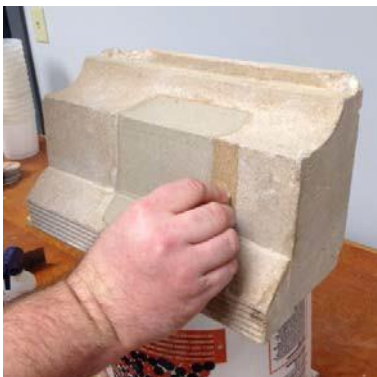
13. & 14. Clean - remove any remaining mortar smears with a damp rubber sponge and clean water. This will prevent any halo effect around patched substrate.
