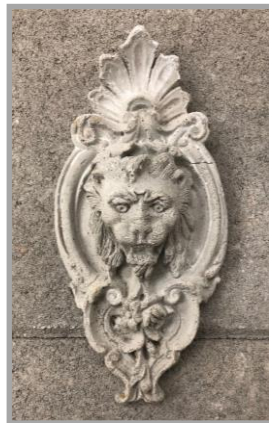
Broken element adhered together
