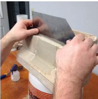
10. Pre-Screed - screed the patching mortar to within 1/4" of the final surface profile. Check for low spots.
