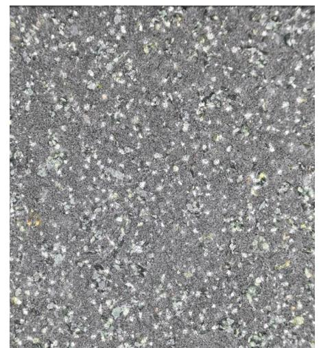
**Burnished** Architectural Series features a smooth-faced concrete masonry unit (CMU) achieved by grinding the surface to reveal the natural beauty of the aggregate within the block. It is available in both structural and veneer options.
