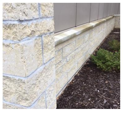
The design of the building required a unique aesthetic element on the concrete masonry portion. Amcon Travertina Series fit the design demand with its multi-dimensional burnished, recessed face texture that mimics the look of travertine stone, but with the economy of a CMU. The block was also selected for this project due to its resemblance to cut-stone.
