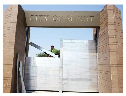
The addition of this large flood wall decreases the community's chance of having to go without clean water in the future. Amcon fabricated the two gateway beams, 378 caps, 40 pier caps, and the large precast City of Minot sign that proudly serves as a city gateway.
