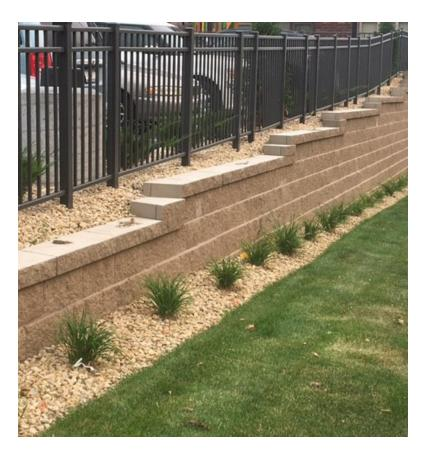
Amcon Concrete Products sales representative Jay Huisken helped with the job. "NorthRock Pro is a new commercial retaining wall product that Amcon provides for use on large commercial applications that can be designed and built with segmental retaining wall units. It is available in 4 stock colors in a straight face. This was a great choice for this project. The material met all expectations and we're very happy with the results." Jay said.
