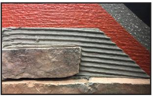
Tenon<sup>™</sup> Waterproofing & Crack Isolation Membrane protects against moisture penetration while providing crack isolation protection
