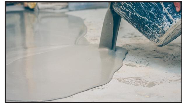
Tenon™ Rapid Patch® Self-Leveling Resurfacer is designed to correct damaged finishes prior to installation of finished flooring or as a wear surfacer for light industrial applications
