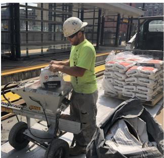
Upon listening to Metro Transit's concerns in conjunction with Kimley-Horn's technical specifications primarily revolving around quality control and repair service life, it was decided to use <a href="Tenon Self-Consolidating Concrete Mix Cl">Tenon Self-Consolidating Concrete Mix Cl</a> with an integral water repellent engineered into the mix.
