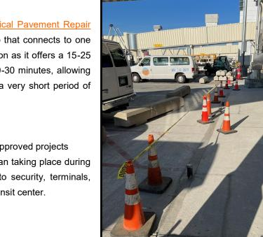
To assist this project, MSP utilized <u>Tenon Critical Pavement Repair</u> (<u>CPR</u>) for pavement repair on a high-use ramp that connects to one of the runways. CPR is perfect for this application as it offers a 15-25 minute initial set time and a final set time of 20-30 minutes, allowing the repaired area to be put back in service in a very short period of time.
