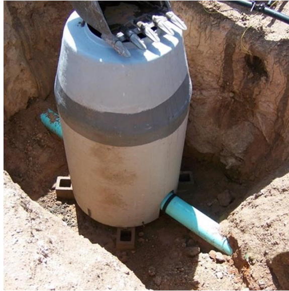
Figure 25. New manhole structure before backfilling.
