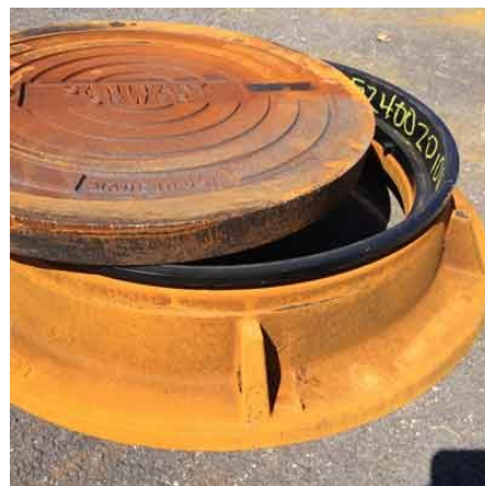
Figure 19. Steel riser ring installed in manhole frame.
