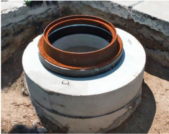
Figure 4. Concrete adjustment rings.
