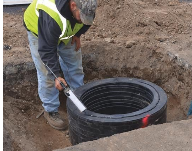
Figure 8. Application of HDPE ring sealant.
