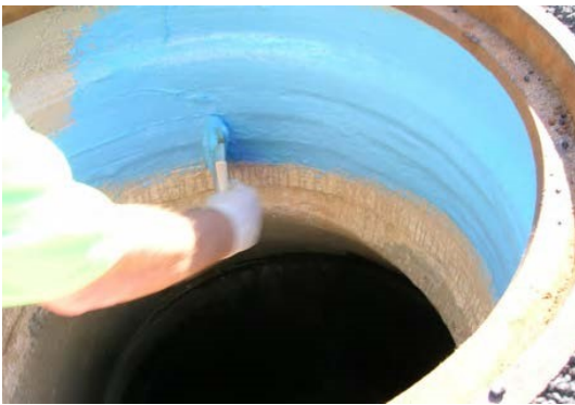
Figure 13. (a) Flex Seal being applied to a manhole chimney interior; (b) Chimney interior after Flex Seal application.
