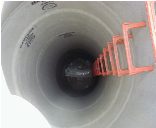
Figure 2. Example of precast concrete (top) doghouse and (bottom) barrel.
