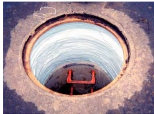
Figure 13. (a) Flex Seal being applied to a manhole chimney interior; (b) Chimney interior after Flex Seal application.
