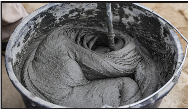
Use Tenon™ Set Retarder in warm weather where extended working time is needed for proper placement
