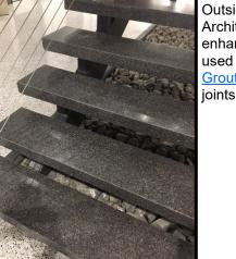
Outside the elevator area, Polished Architectural Veneer was added to enhance the aesthetics. The installers used <a href="ProSpec Stone Veneer Joint Grout">ProSpec Stone Veneer Joint Grout</a> by TCC Materials to grout the joints.
