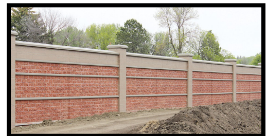
Image of floodwall at Water Treatment Facility. 2017. Minot Daily News https://www.minotdailynews.com/news/local-news/2017/05/stain-being-applied-to-water-treatment-plant-floodwalls/
