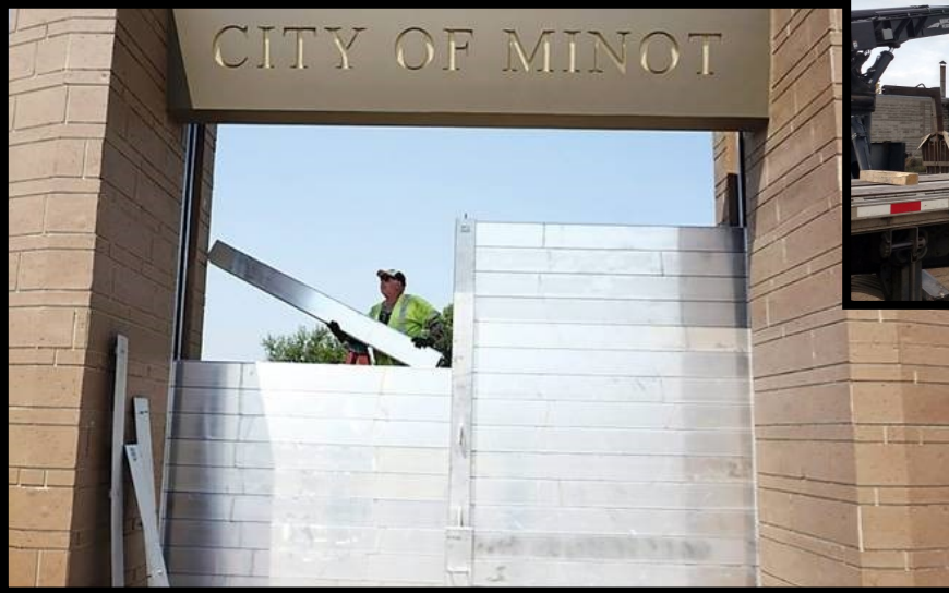
Schramm, Jill. Image of worker assembling flood wall. 2017. Minot Daily News. https://www.minotdailynews.com/news/local-news/2017/07/city-crews-train-on-16th-street-flood-wall-closure/
