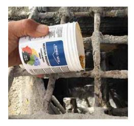
**STEP 1** Using a mechanical batch mixer to ensure mortar uniformity and good workability, add the minimum amount of clean, potable water to achieve the desired consistency. With the mixer running, empty the SPEC MIX Mortar Color container into the mixing water.
