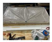
**7.** Once 18-24 hours have passed, remove the plastic from the countertop surface and remove all the screws holding the form together. The countertop is still fragile, so be careful when removing forms. If necessary, use small wooden shims to help remove the side panels of the form. Finally, gently remove the bottom of the base.
