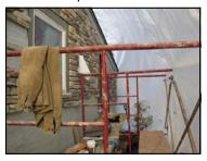
**Proactive measures** should be taken to avoid problems occurring from cold weather. Choosing the correct materials, heating materials, building partial or full enclosures, and using admixtures are a few ways to combat cold weather conditions.
