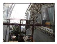
In cold weather the cement hydration process continues for an extended time period. Heating and protection are required to ensure that masonry surfaces under construction do not extract excessive heat from the mortar and grout. When the mean daily temperature is below 40°F (4.4°C), protective measures are required.
