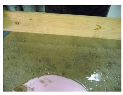
**8.** Vibrate the form by tapping with a rubber mallet around all the edges or by using a palm sander without any paper on it. This is an important step to minimize pinholes in the countertop surface. Screed of any excess material with a 2"x4".
