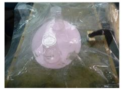
**9.** After the material in the form has begun to take a set, normally 1 hour, snip off the wire ties holding the wire mesh just below the surface of the countertop mix. If needed, screed the back off, using a 2" x 4" moving it in a sawing type movement against the top of the side forms. Cover the countertop mix with plastic and allow it to cure 18-24 hours.
