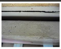
**10.** Remove the plastic from the countertop surface and remove all the screws holding the form together. The countertop will still be very fragile so use care in removing forms. If necessary, use small wooded shims to help remove the sides of the form. Put down some small pieces of foam next to the base of the form. Then hold the base of the form and the countertop, lift the countertop onto the foam in a vertical position. Gently remove the bottom of the base.
