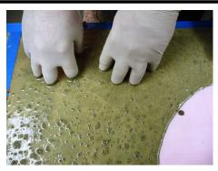
**7.** Fill the countertop form with the mixture making sure it fills in around any reinforcement and around all cutouts. Knead the material with your hands to assure the material is evenly spread throughout the mold and to eliminate air holes. Gloves should be worn for this process.
