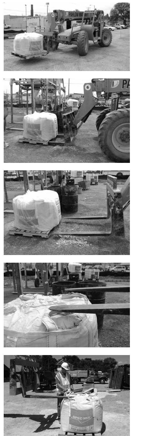
1. When transporting bulk bags, only move the bag while seated on a pallet. The boom of the fork truck should be fully retracted. Do not transport bulk bags around the jobsite suspended from its lifting straps.
