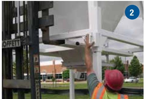
**Step 1:** To erect the silo on site, make sure the ground is dry, level and compacted. With a 26-foot, 4,500 lb capacity standard forklift, insert the forks of the lift into the silo's fork pockets and raise the unit to the desired height. Four heights are available.
