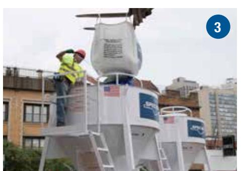
**Step 3:** The bulk bags are easily loaded into the silo by inserting the forks through the bag's reinforced loops. Once the bag is above the silo and in position over the upper dust shroud, the laborer standing on the safety platform can release the bag's double discharge chutes.
