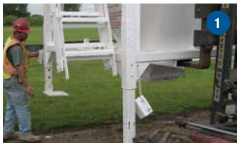
A double batch of material is made in 5 minutes or less without straining the laborer's or compromising the integrity of the mix. No electricity or pressurized water source is needed, just a standard mechanical batch mixer. The silo is transportable. As the job progresses, the crew and silo mixing station follows.
