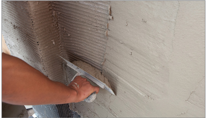
Application of proprietary, preblended, shrinkage compensated basecoat
