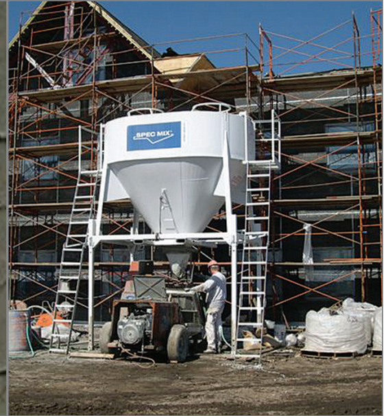
SPEC MIX silo system improves production and mix consistency and eliminates the disposal of wasted sand and bagged goods
