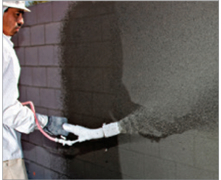
SPEC MIX FBC Stucco is engineered for gun-applied basecoat in one- and three-coat wall systems
