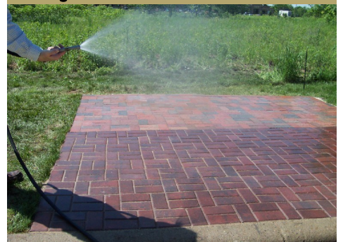
Wetting of Joints
