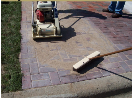
Filling of Joints
