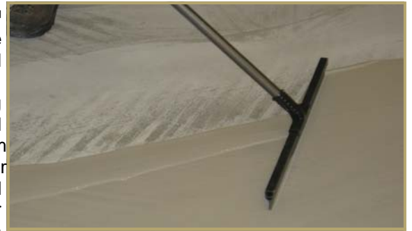
Example 2: Apply Akonakote™ using a stiff-edge blade
