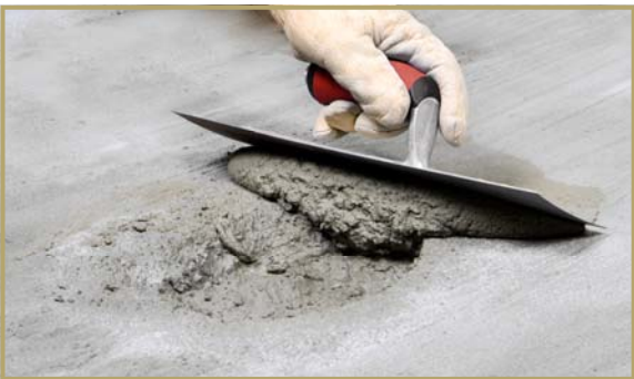
Example 1: Repair deeper blemishes with Rapid Patch™
