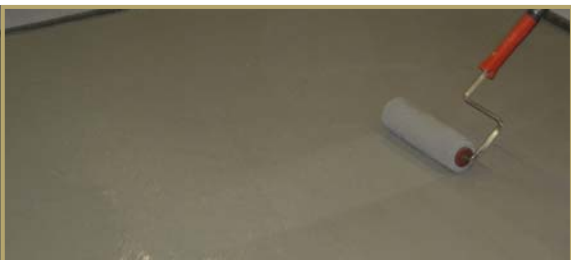
Example 4: Apply sealer using a roller
