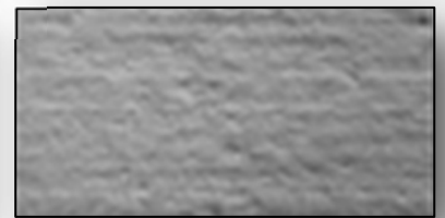
CSP 4 (light scarification)
