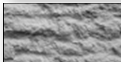
CSP 9 (heavy scarification)
