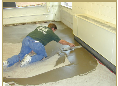
Figure 2: Applying with trowel
