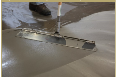
Figure 3: Applying with stiff-edge blade
