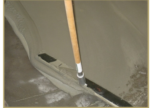
Application of Pourable Concrete Patch
