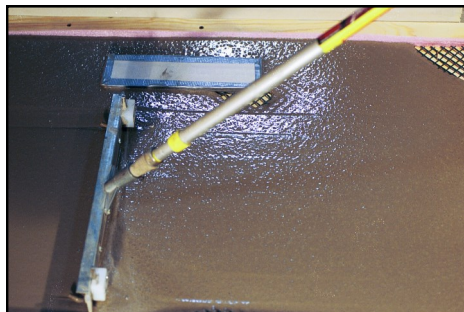
A gauge rake designed for underlayments may be helpful for larger areas
