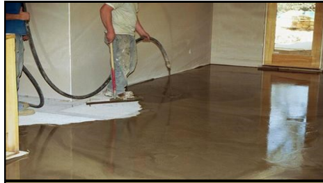
Applying Self-Leveling Floor Underlayment Cement thru a pump
